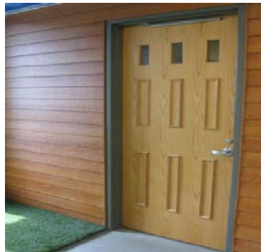
Mock house – front door
